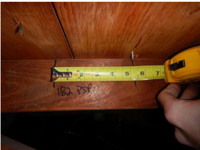
Roof Deck Attachment
