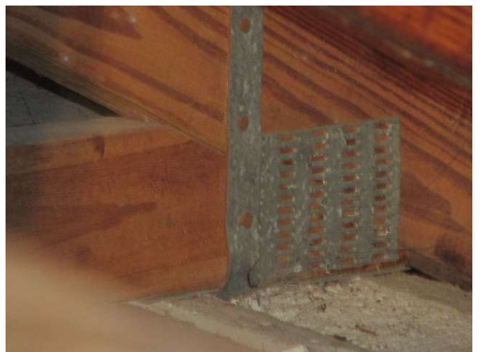
Roof to Wall Attachment
