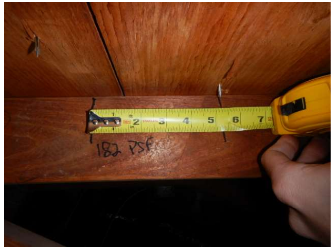
Roof Deck Attachment
