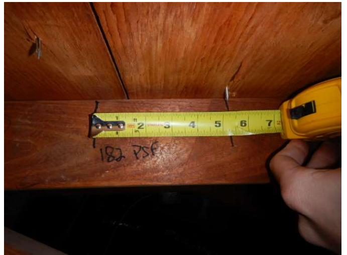
Roof Deck Attachment
