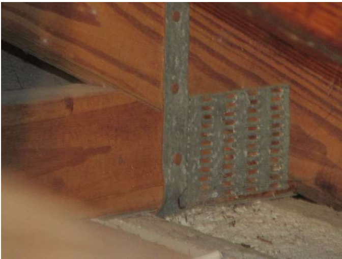
Roof to Wall Attachment
